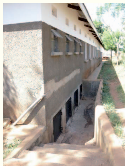
Picture 5: Emptying doors at the back of the building (Kitgum, Uganda).
