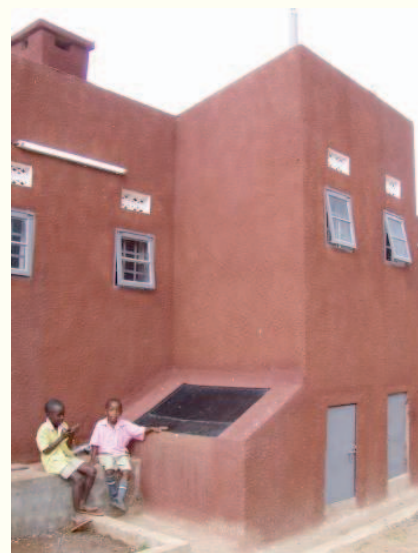
Picture 7: UDDT from the backside of the house (Naggalama, Uganda).
