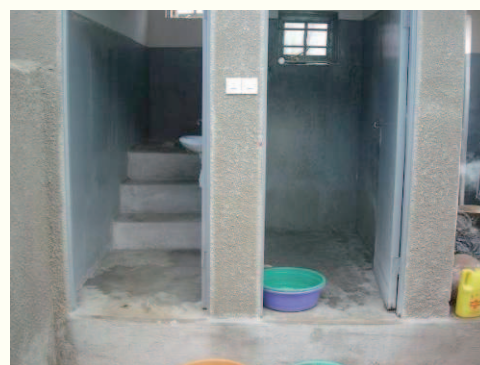
Picture 6: UDDT and bathroom attached to a staff house (Naggalama, Uganda).
