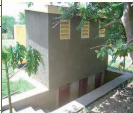
Picture 1: UDDT with underground faecal collection chambers at KTC (Kitgum, Uganda).
