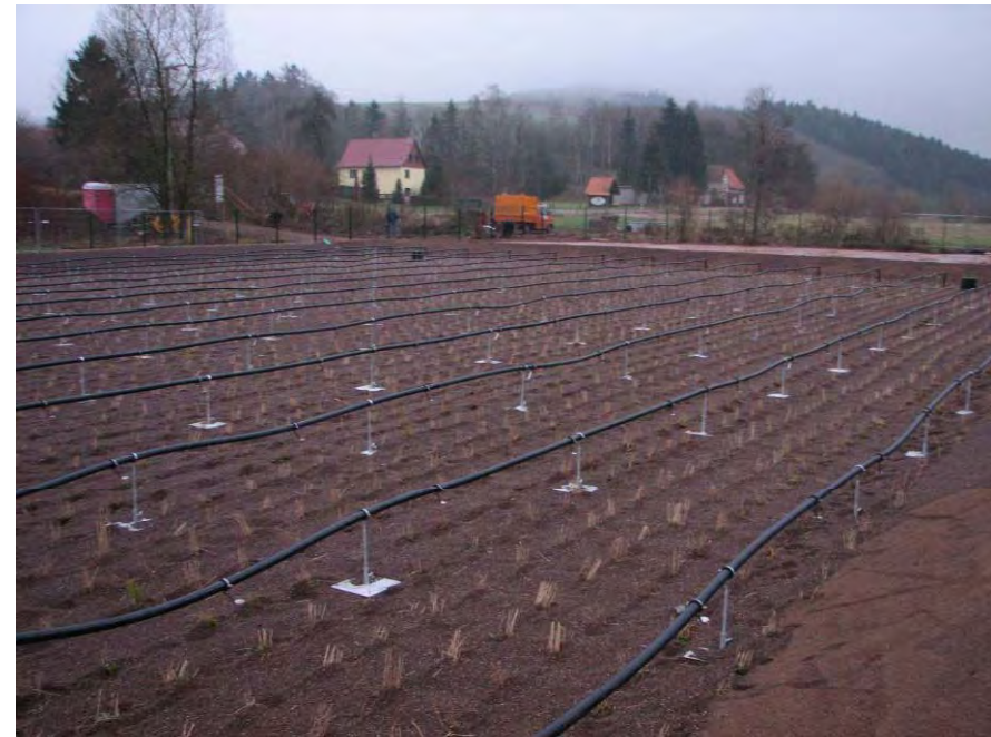
Wastewater distribution system
