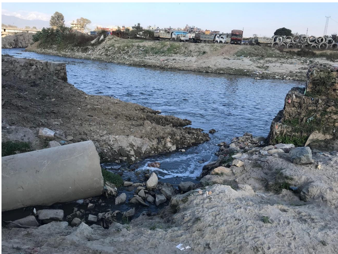
Figure 3: Wastewater and supernatant discharged into Bagmati River untreated.
