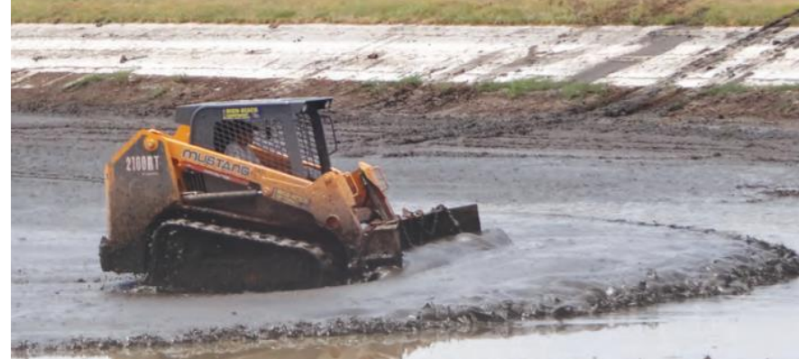
Figure A6.8: Tractor pushing sludge in pond
