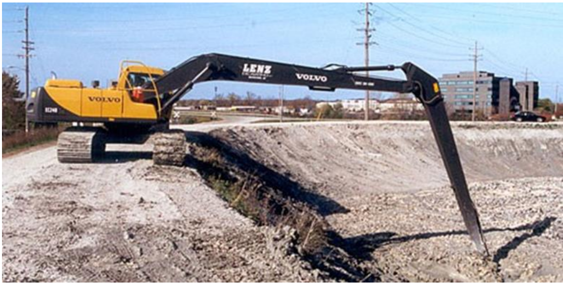
Figure A6.6: Track hoe used for sludge removal from pond cell
