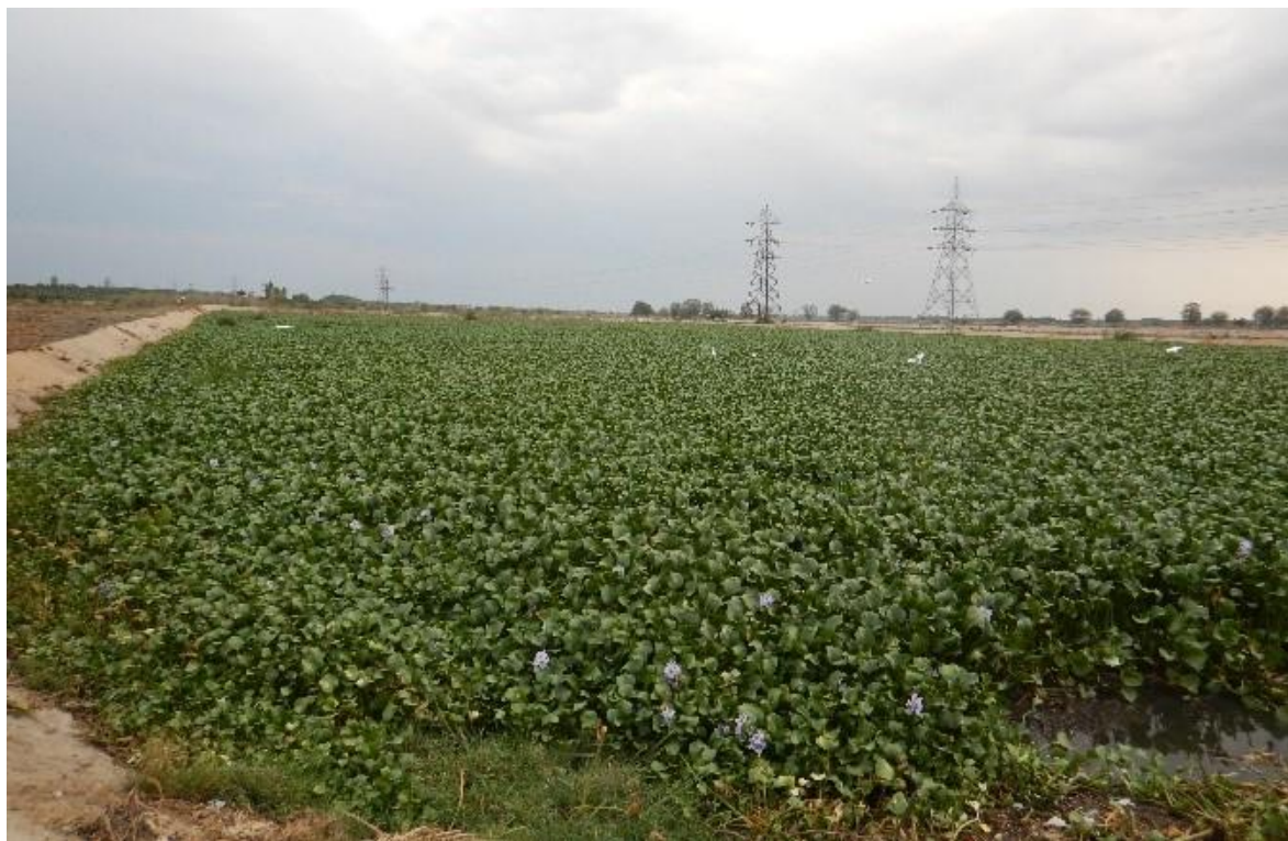
Figure 2.9: Anaerobic Pond with Surface vegetation
