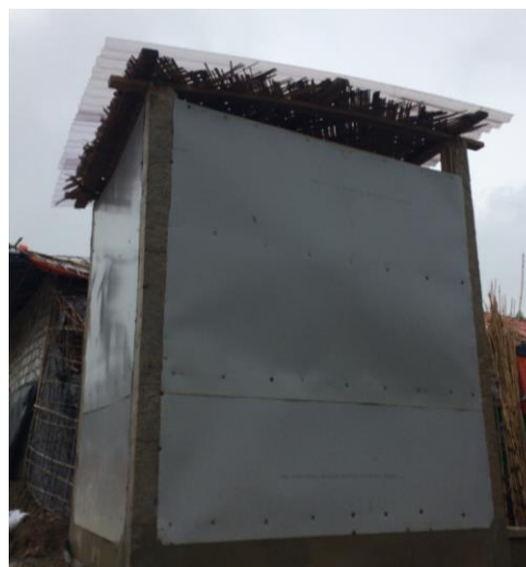
Figure 5: Transparent Roof with Wood
