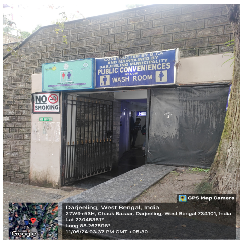
Figure 3: Public Toilet near Mahakal temple (Source: Shatabdi/NIUA/2024).
