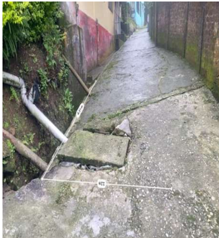
Figure 16: Community Septic tank in Ward 11 (Source: Sachin/NIUA/2024).
