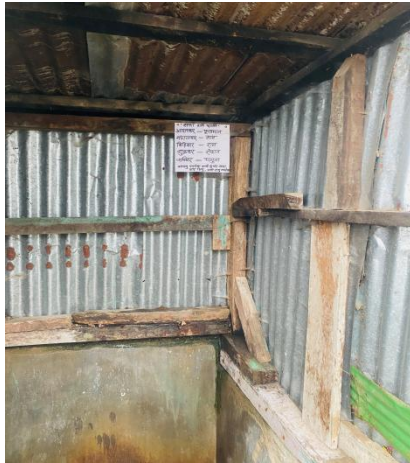
Figure 5: Shared household toilet in Ward 14 (Source: Sumit/NIUA/2024).
