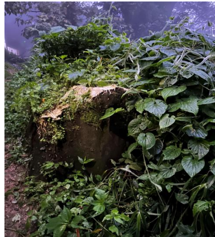
Figure 17: Abandoned Community Septic Tank in Bhutia Busty (Source: Anant/NIUA/2024).
